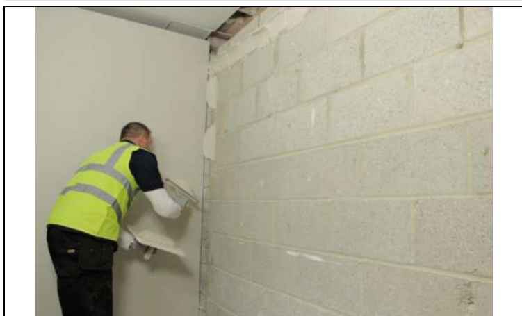
Figure 2 Direct bonding to wall
