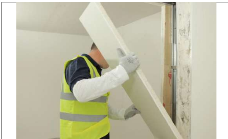
Figure 4 Window reveal installation
